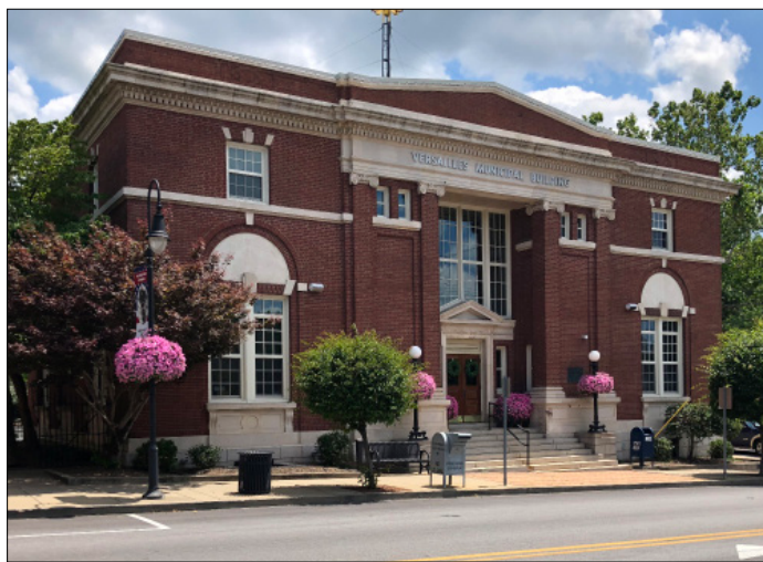
Versailles Municipal Water and Sewer Department
